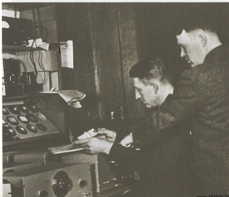
Dave Packard (seated) and Bill Hewlett run final production tests on a shipment of 200A audio oscillators, the product that put them in business in 1939. The shipment may possibly have been the order of eight instruments that went to Walt Disney Studios in Hollywood for production of "Fantasia." Site of the above scene was the garage located behind the home rented by the Packards at 367 Addison Avenue, Palo Alto. Lucile Packard and Flora Hewlett, the wives of the partners, were important contributors to the young company during these early years, pitching in on administrative and even production tasks.
